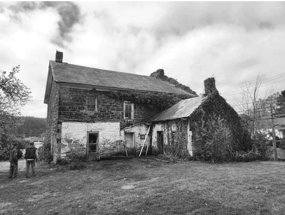
Above: The back of the jail had ivy issues as well as paint issues with the paint being manually removed by hand so as not to further deteriorate the mortar of the stone.
