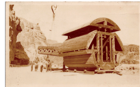
Above & Below: This "animal" postcard depicts a construction machine designed and built to fill 18 feet diameter tunnels with concrete. Unknown date and location, but this RPPC is valued at $34.
